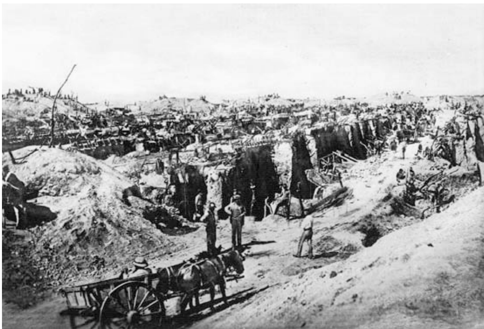
Only linking roadways remained
