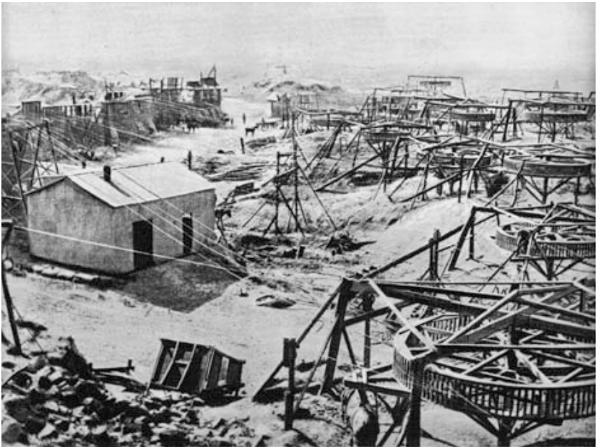
Horse-driven winches at the Kimberley mine
