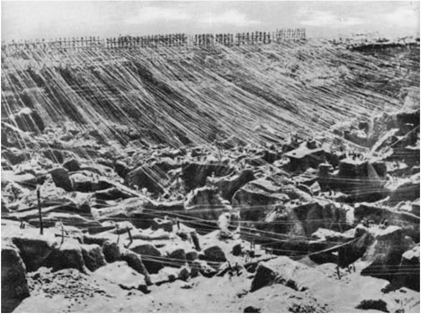
Cables for the mining bins
