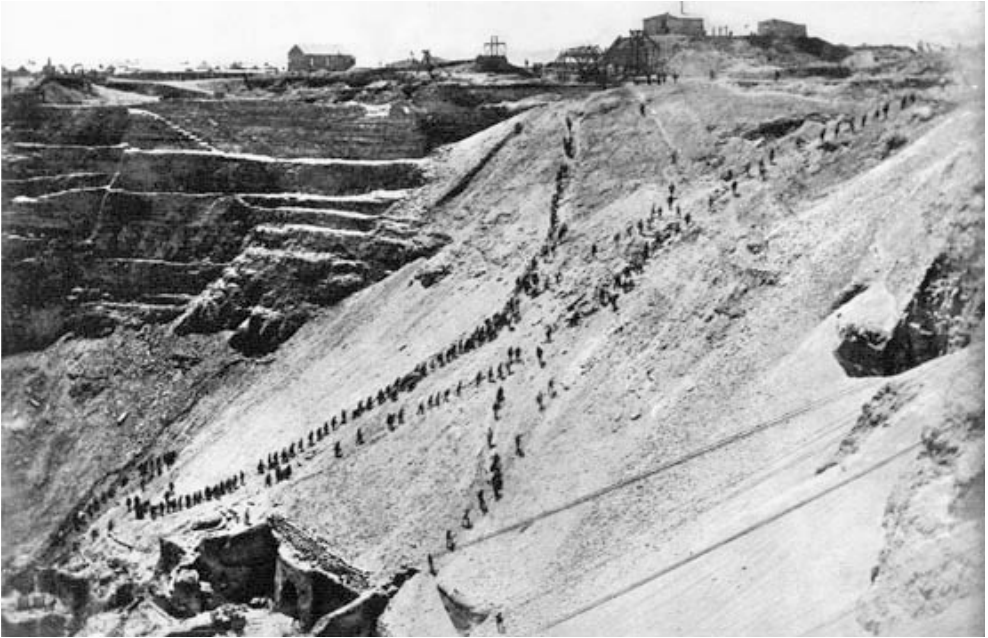
End of the working day
