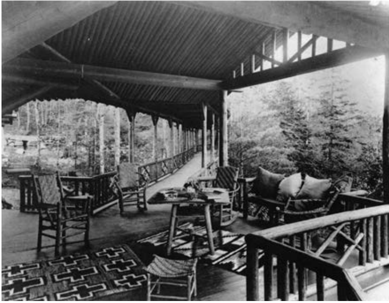
Exterior view of one of the walkways between the houses
