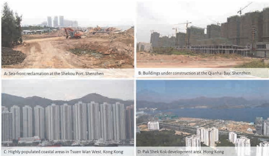
Figure 2: Photographs showing the rapid development and urbanization in the low coastal areas of the PRD. Source: Photos taken by Liang E. Yang in November and December, 2011.
